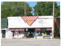
Milda's Corner Store 9901 Townline Road Union Pier
