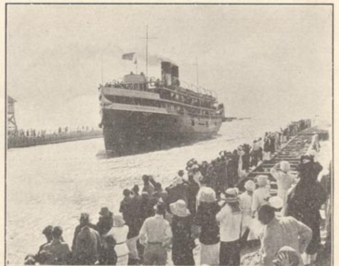
Harbor Entrance and Piers at South Haven
