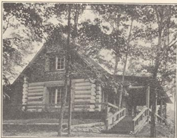
"In All the World OLD TRAIL TAVERN No Place Like This"
