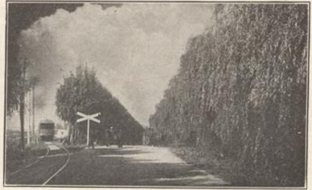
Junction of the Grand Highway with the West Michigan Pike
